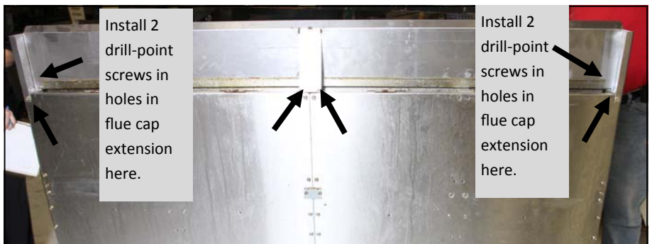
Figures 3,4: Attach flue cap extension with removed screws and provided drill-point screws at positions indicated by arrows. A flange (see photo, right) on the flue cap extension grips the existing flue cap behind the middle brace.
